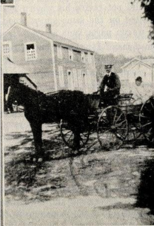
Figure 11. Tenement House in Factory Village
