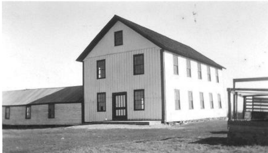
Figure 2. Middlefield Fair exhibit hall. Date unknown, taken after the flat roof was covered with a peak to prevent snow damage, and before electricity came to the fair in the early 1930s. 48
