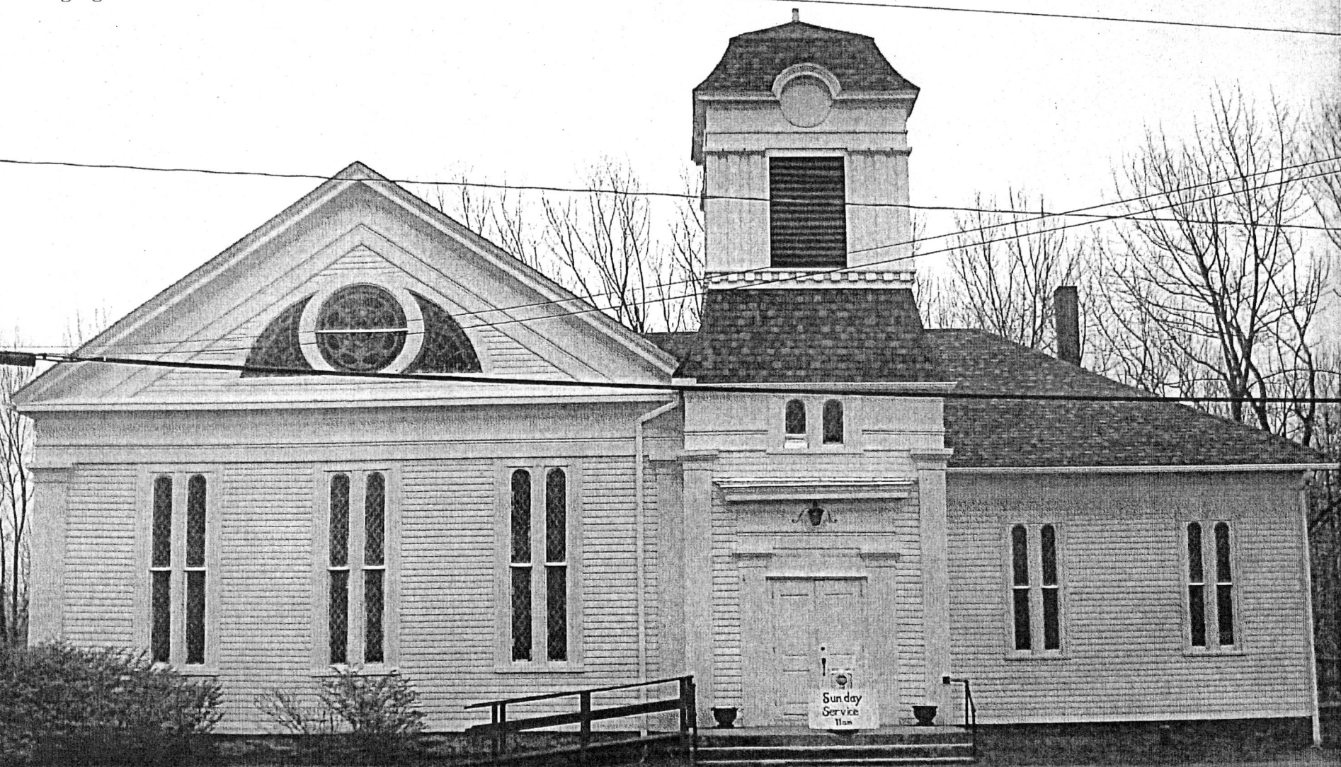
MIDDLEFIELD CENTER HD: Congregational Church, 167 Skyline Trail
