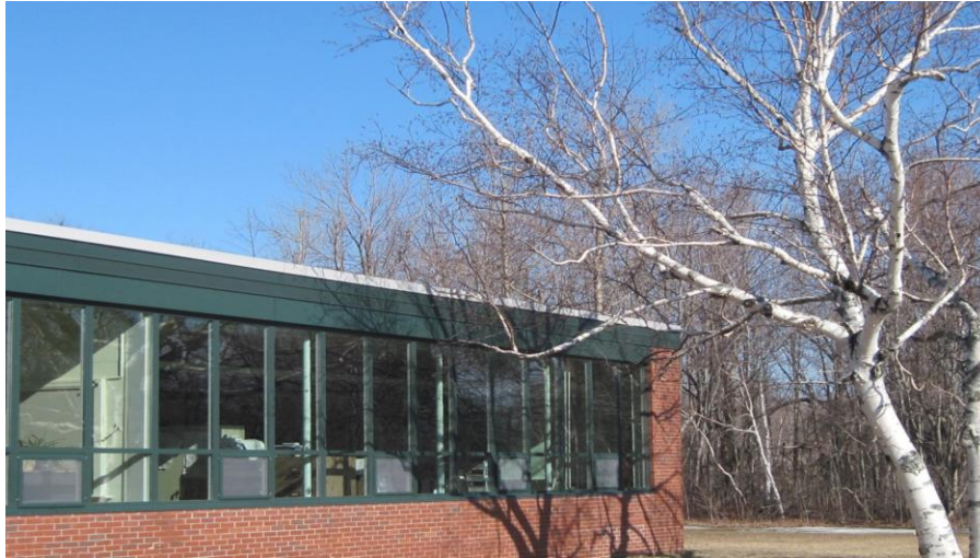
New windows at the Town Hall
